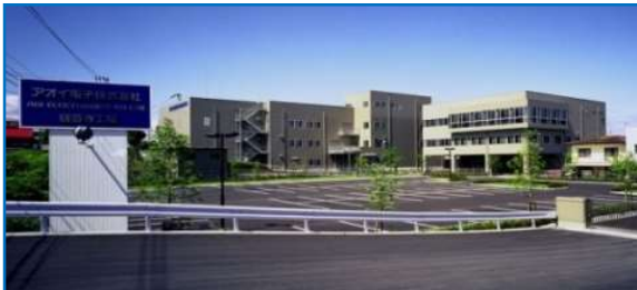
■ AOI-ELECTRONICS KANONJI PLANT
